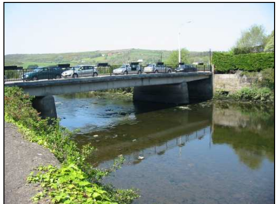
John F Kennedy Bridge
