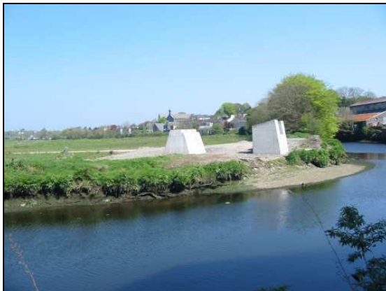
Abutments for New Footbridge
