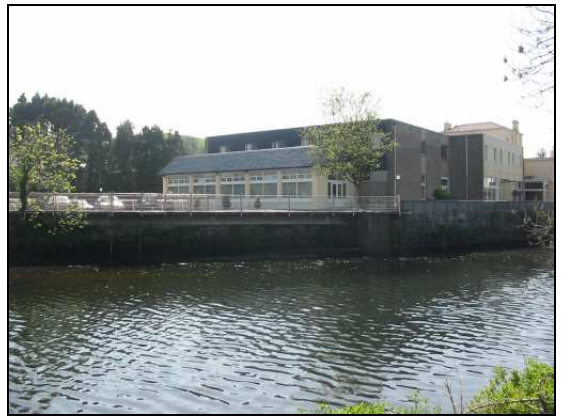
Cantilevered Walkway at Hotel
