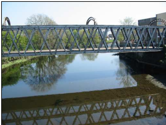
Cast Iron Railway Bridge
